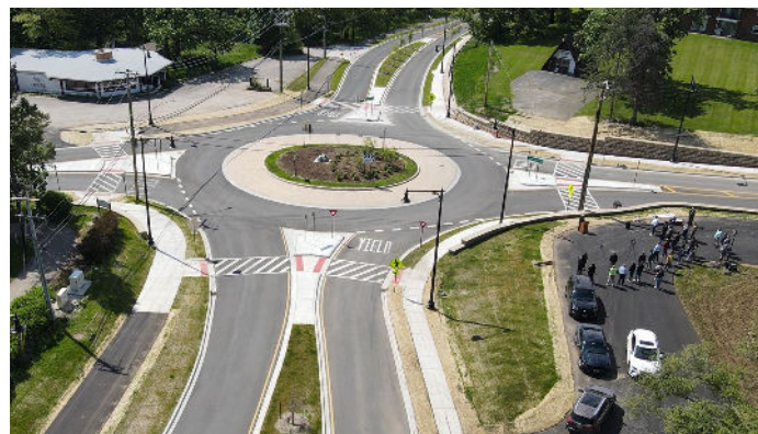
Algonquin Main Street Reconstruction Project
